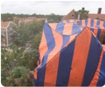
A large, multi-unit structure tented for fumigation with Vikane.
